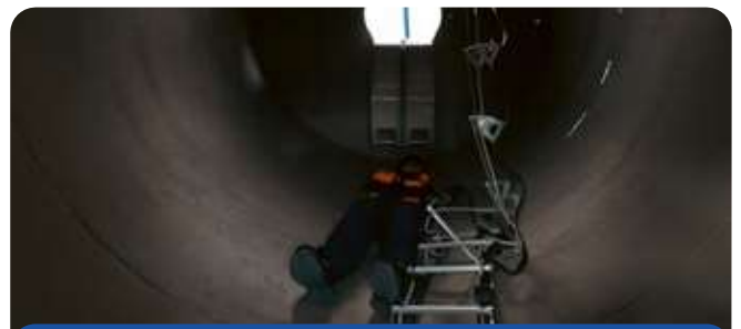
Confined space cistern
