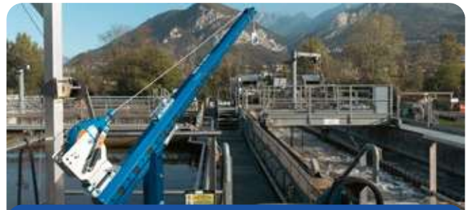
Confined space tank
