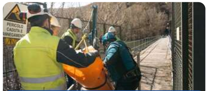
Confined space dam
